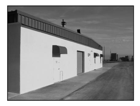
Figure 2. Front laboratory limewash, not pigmented.
