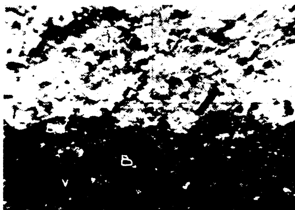
c. Surface photo of 1:2:7 cement, lime, sand mortar (age 37 years) which exhibits good contact in spite of rough brick surface (reflected light, 20x magnification).
